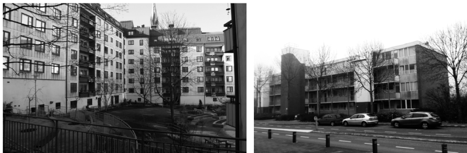
Figure 4. Housing buildings built using reused precast panels: the Gothenburg (left) and the Middelburg (right) [6]
