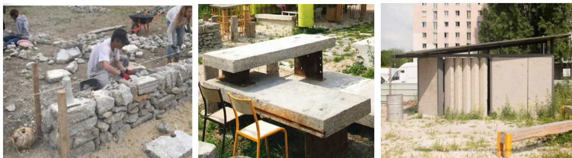
Figure 5. Reuse of concrete in La Fabrique du Clos by Bellastock [7]
