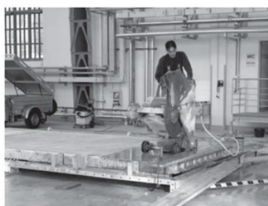
Figure 3. Processing of the de-mounted components with a concrete saw.
