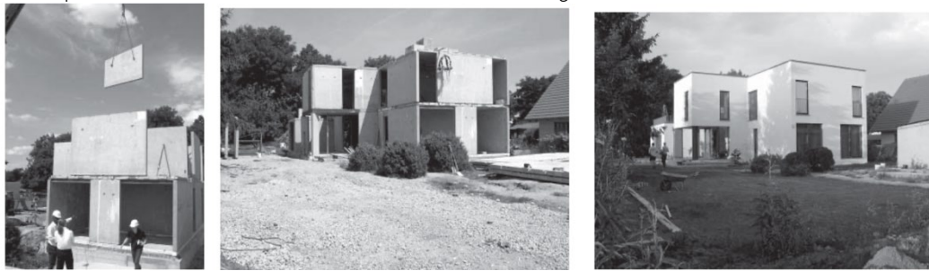
Figure 3. First pilot house reusing WBS70 concrete panels. [5]
